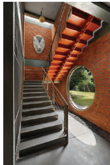
► The beautifully crafted staircase which connects to the upper floor is made of 10mm folded metal plates with two open-to-sky slits in the slab which imparts a magical effect to the walls and enhances the ceramic art on one wall and a desi painting in kalamkari art on the other wall. A round cut-out in the staircase wall connects the space visually to the greenery outside.
