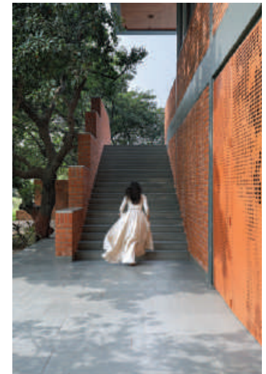
▶ A part of the south facing façade & the steps leading to the deck area on the west side adjoining the infinity swimming pool.
