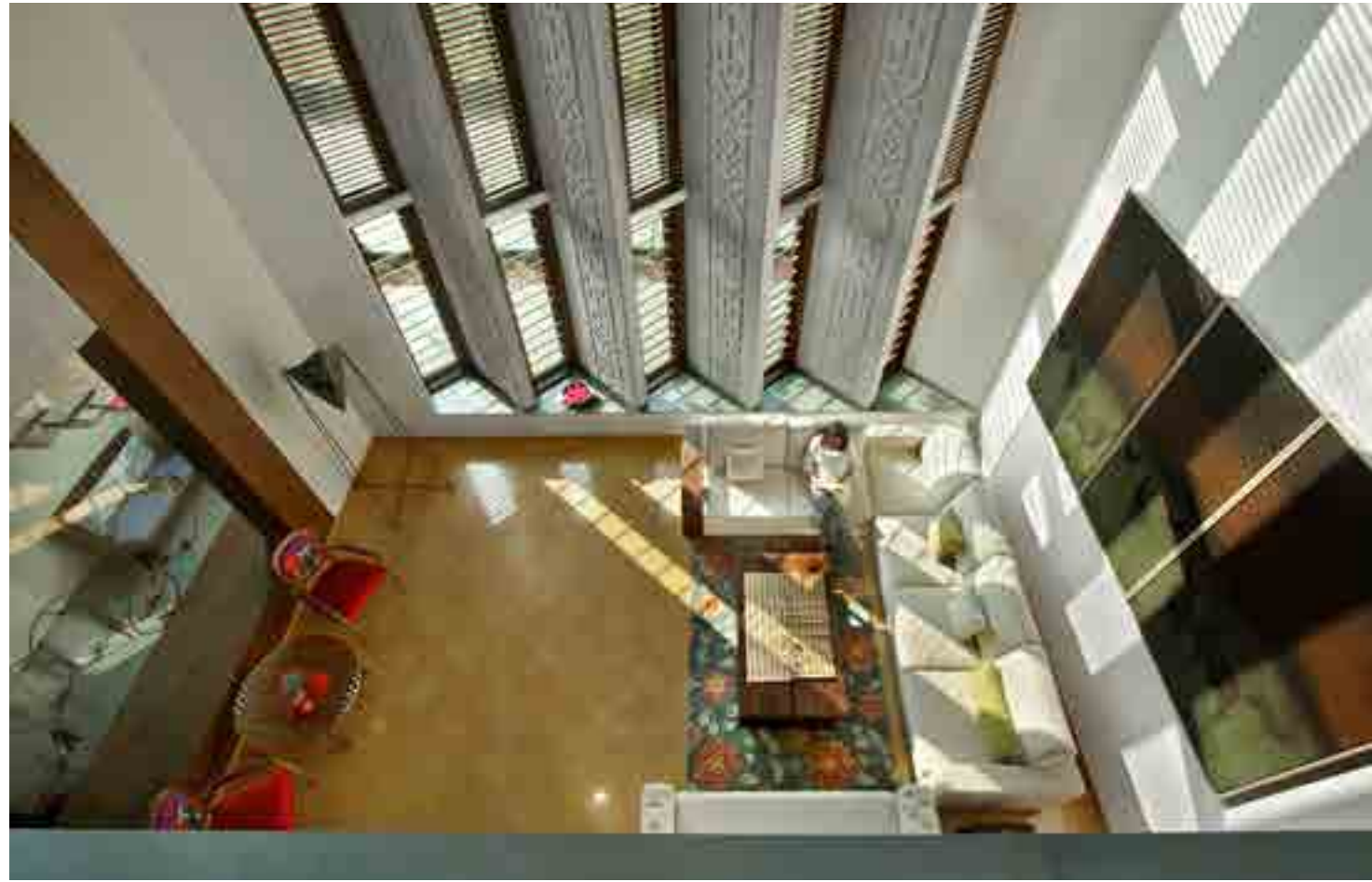
Tall, bold concrete fins guard the west façade with intricate design details carved on their surface.
