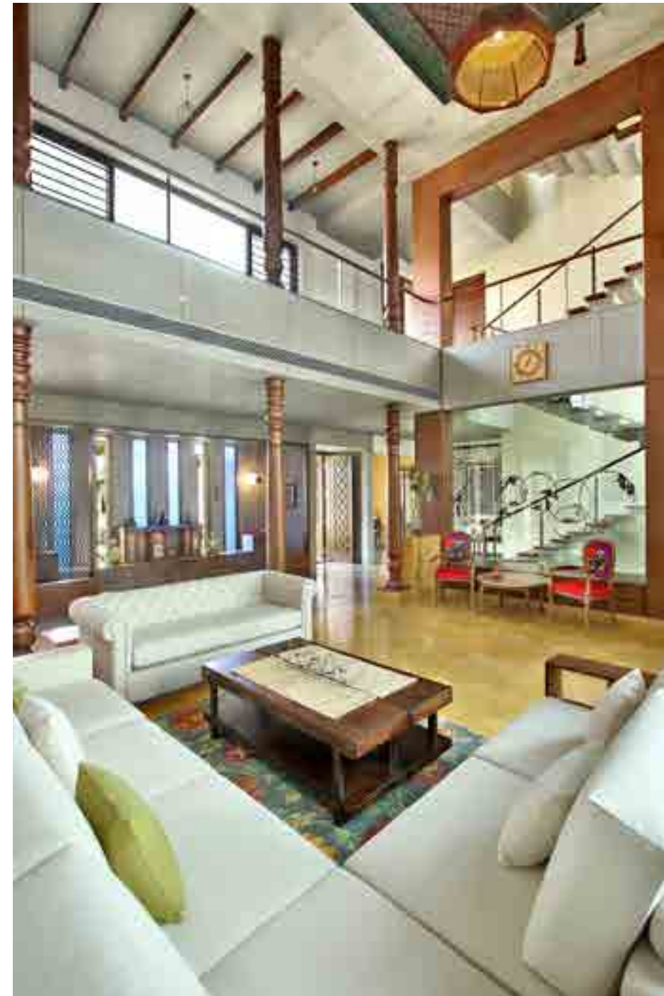
The double height is capped by an exposed RCC slab layered with a specifically customized wooden panel with brass inlay sourced from Anjana handicrafts, Ahmadabad.
