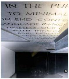
Before using exposed concrete elsewhere on sites, we practised at our own office, along with an engraved script which speaks about our firm's motto. It is an exposed concrete's slab, with beautiful engraving. Self-flowing concrete was taken into account for this slab. After the success of this experiment, our boundary of limitation widened and we became more confident about adapting the new ideas and techniques.
